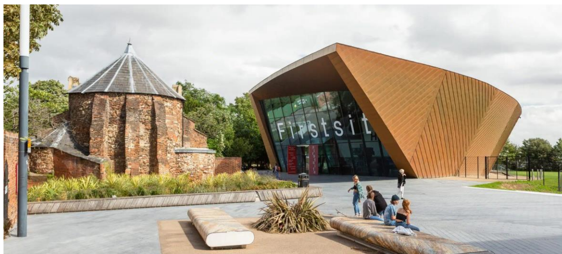
IMG 7 – Firstsite Building 7
